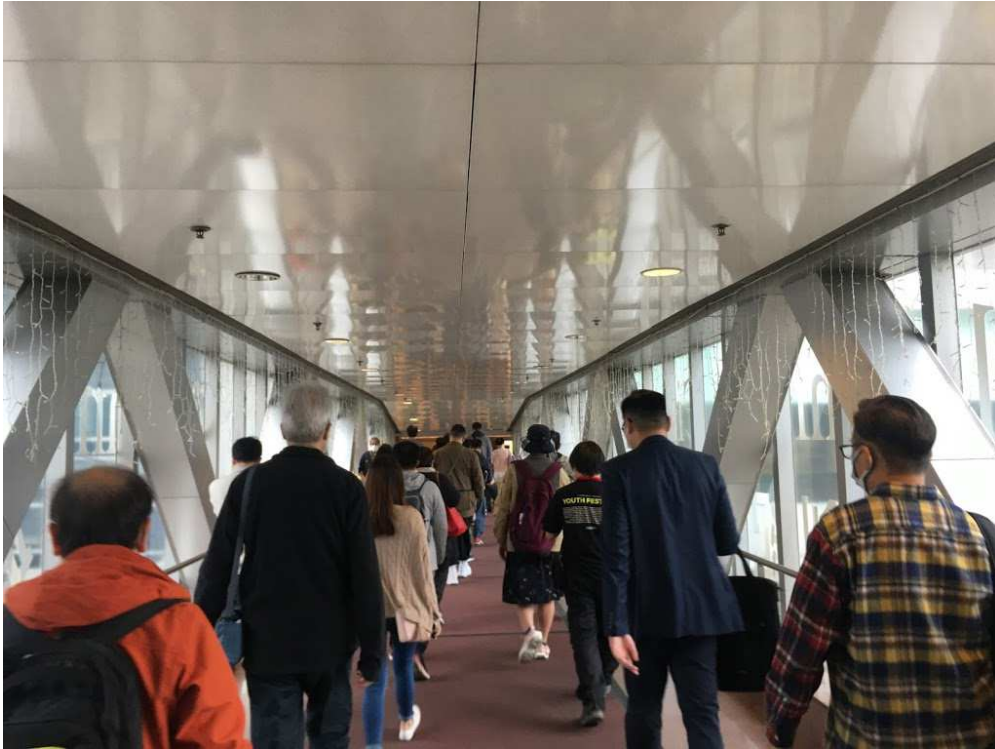
Millennium City 2 & 3 footbridge
